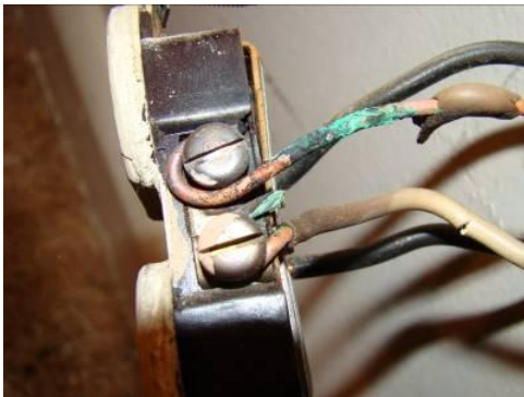
Figure 8: Floating neutral
